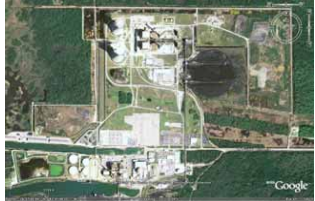
Fig. 4. The Progress Energy Crystal River Facility with 4 Pulverized Coal Plants and 1 Nuclear Plant.
